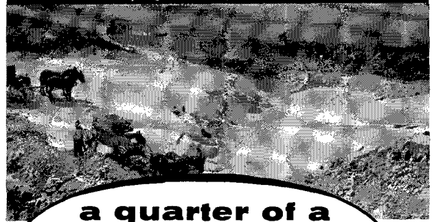
1930 Quarrying for first plant—Walteria
